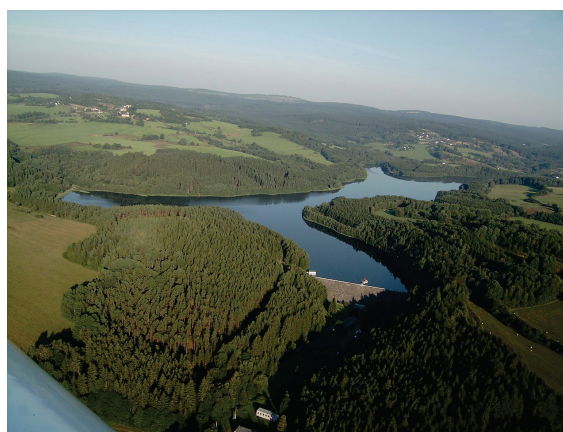
Lučina water reservoir (Source: https://cs.wikipedia.org )
