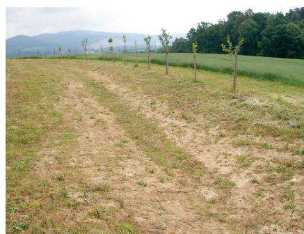
Retention swale (source: http://www.zabreh.cz )
